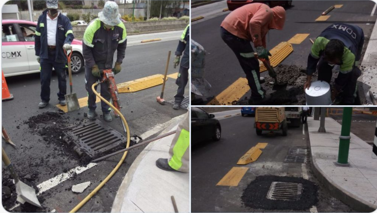
IMPROVEMENT OF SEWAGE ACCESORIES
